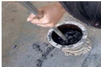
Fig. No: 6.4.2 A) Placing Of Concrete In Mould
